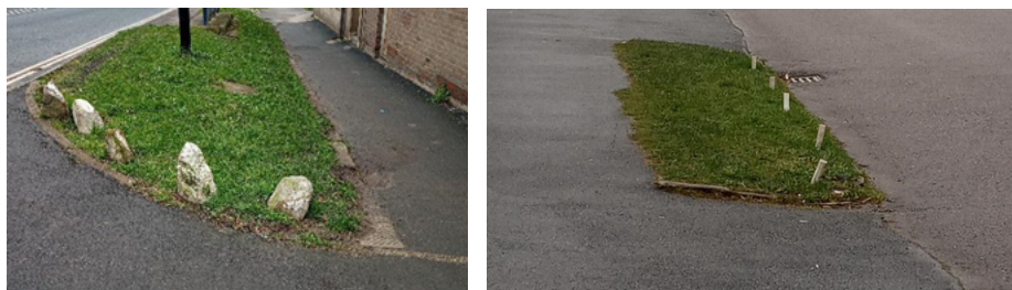
Examples of resident installed verge protection measures to prevent parking
